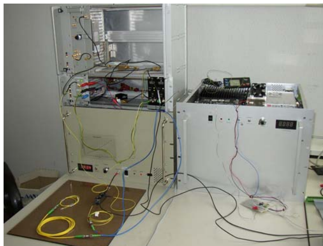
Figure 9.1.2: Very first FO distribution system test.
