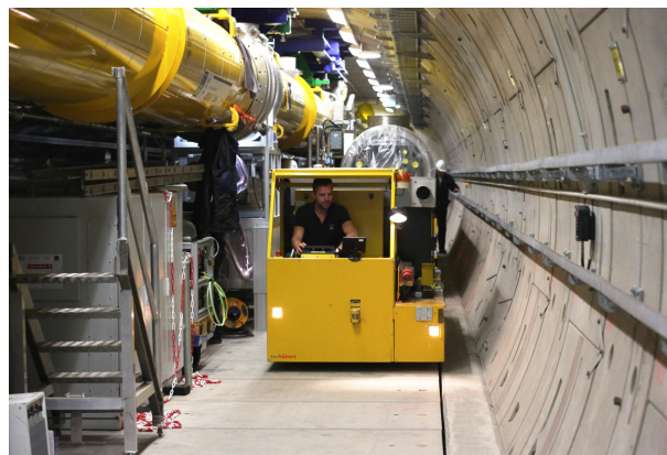
Figure 2: Cryomodule transport into the XFEL tunnel.
